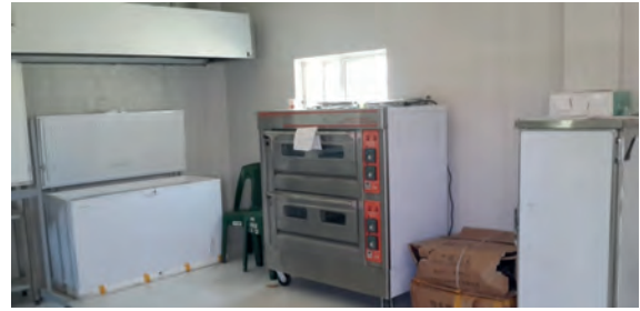
Figure 36 Food production kitchen at JWQTS
